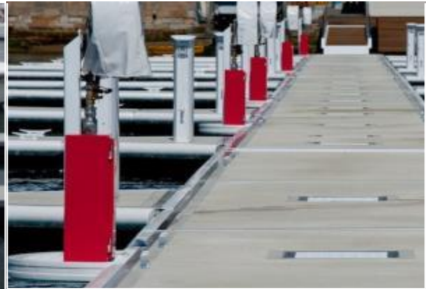
Fire extinguisher box & fire hose
