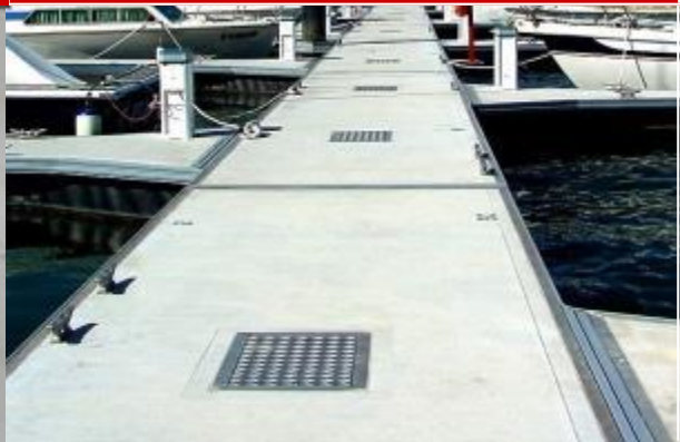
Service pits with internal conduits
